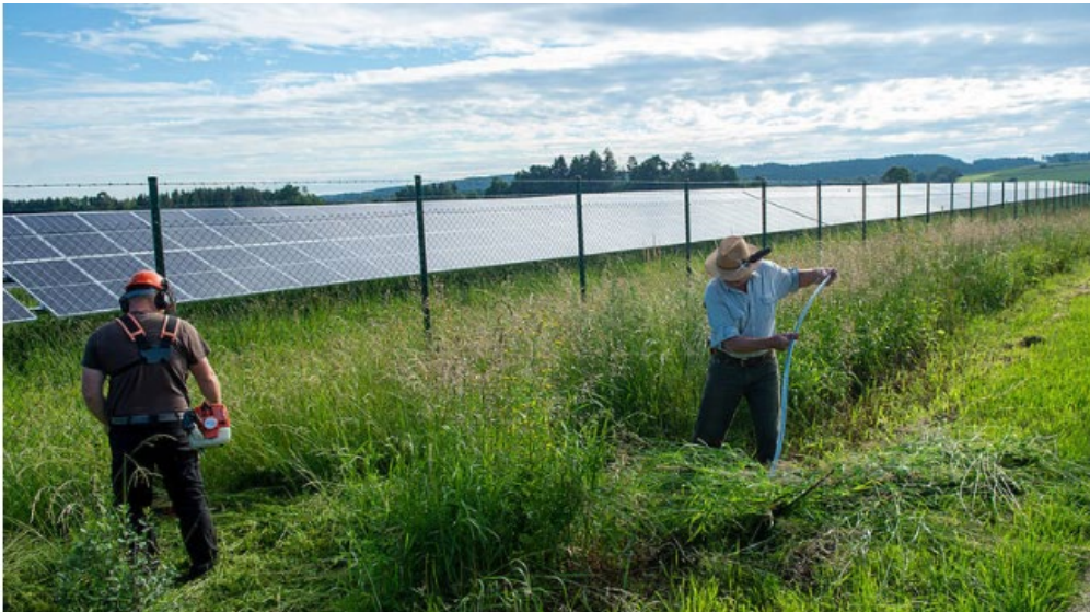
Typical panels and fencing
